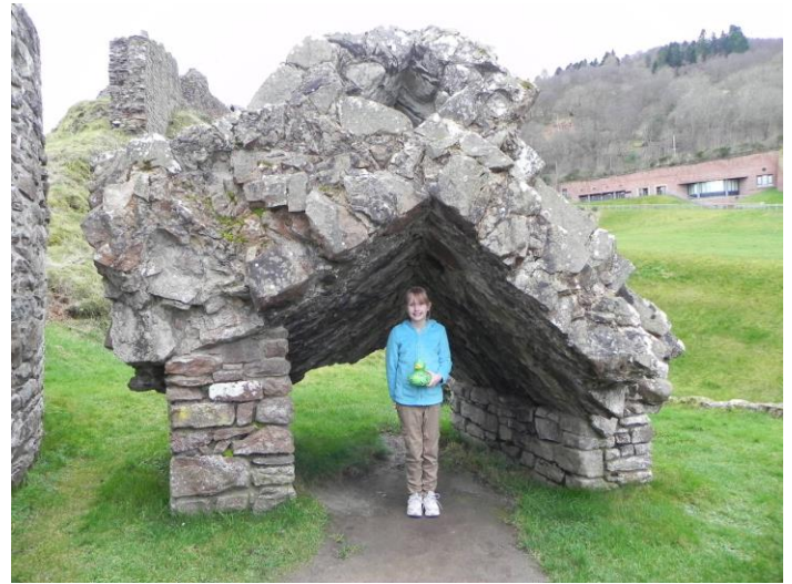
Photo features El Wallace, 2012, inside the remnant of the gatehouse.
